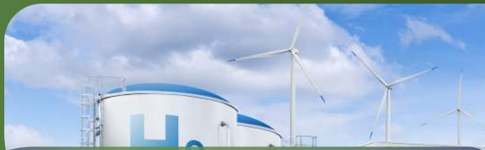
Commencement of construction work on a number of renewable energy and green hydrogen projects in Duqm
