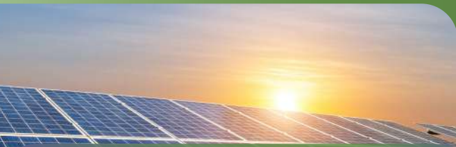
Operation of Manah 1 and Manah 2 solar power stations
